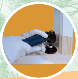
1. Remove paint & dirt
