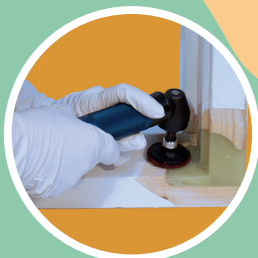
6. Sand finished repair
