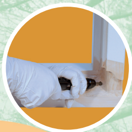
2. Remove all decay
